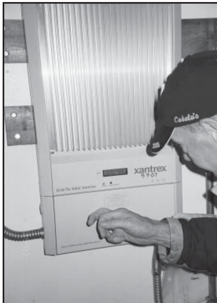
Father Joseph Hemmer, O.F.M., checks the Xantrex GT 2.8 inverter by simply tapping below the digital display.
